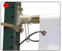
Use the other safety pin and fasten it to the zip tie and the safety pin holding the mount to the pole. This will make sure the graphic doesn't slide off.
