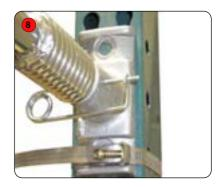
Close the safety pin and the finished pole and pole mount should look like this.
